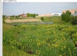
When new business parks were created on an existing site, a **shared infiltration solution** was implemented. It consists of creating shared infiltration basins. The treated water leaving the retention basins is then directed to infiltration areas consisting of a long strip of gravel.
