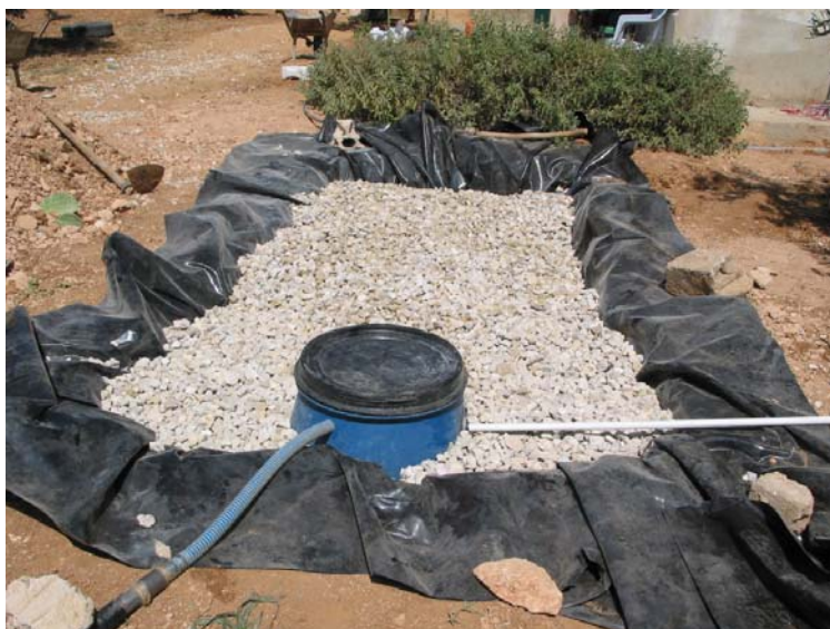
Figure 3: Installed confined trench greywater system.
