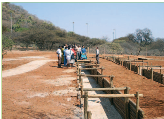
Training unit for the laying out of mains
