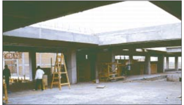
The construction site: the educational building
