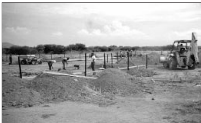
Construction of the new documentary centre has just begun
