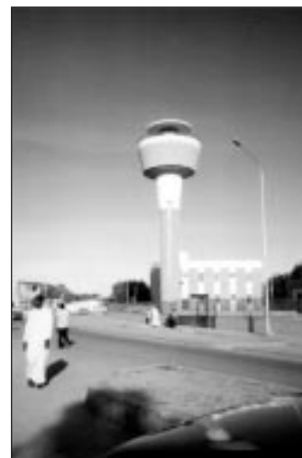
A water reservoir in N'Djamena
