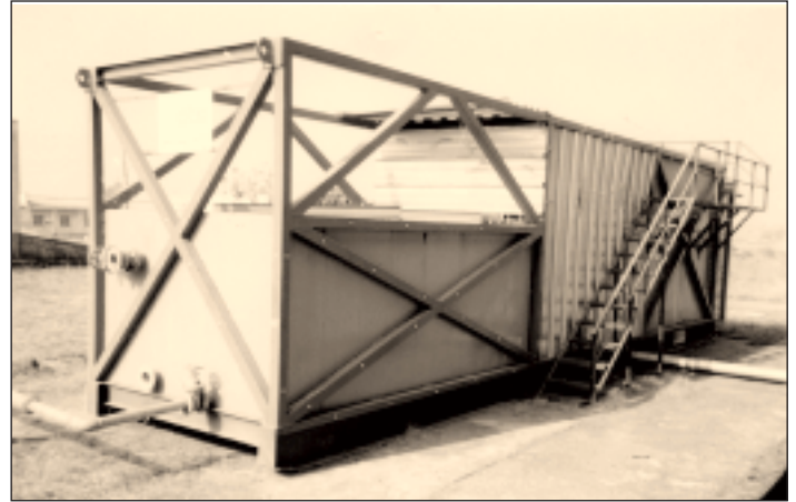
OTV's pilot unit for drinking water production
