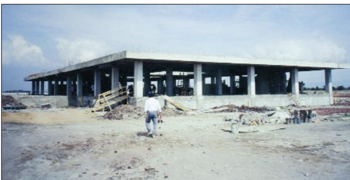
Texcoco, the construction site viewed from outside
