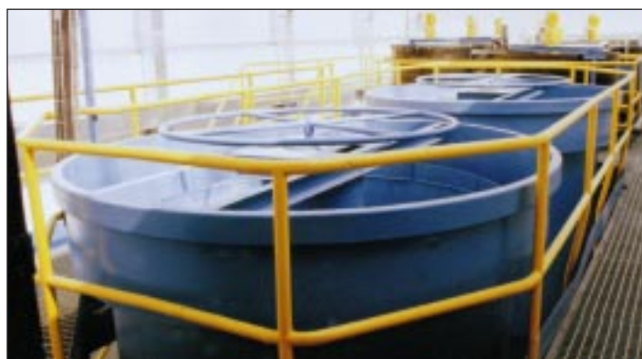
The STEREAU's wastewater treatment pilot unit
