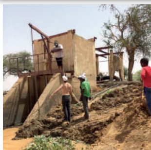
Installation of the station in Kollo
