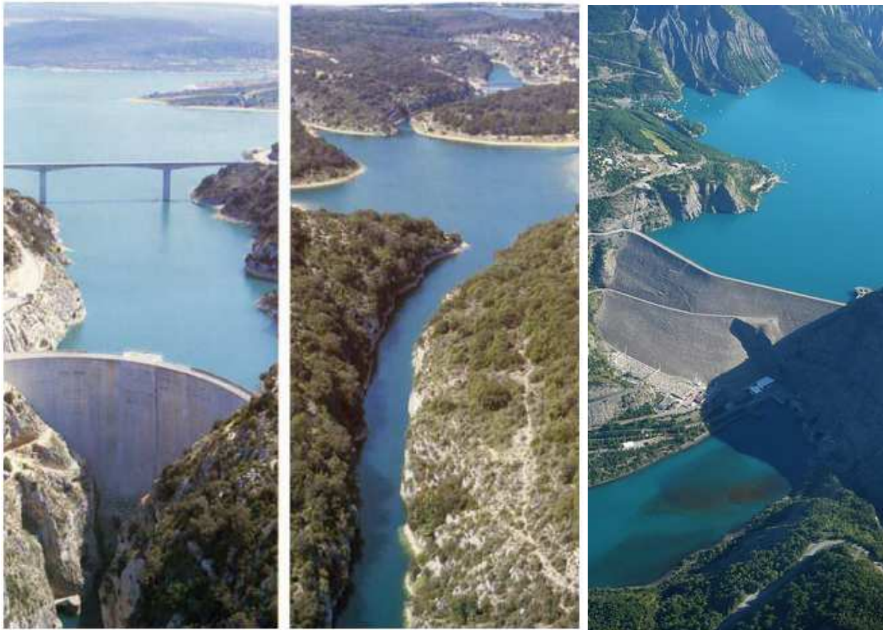
Figure 17: the Sainte-Croix dam on the Verdon (SCP) and Serre-Ponçon dam on the Durance (C. Ben)
