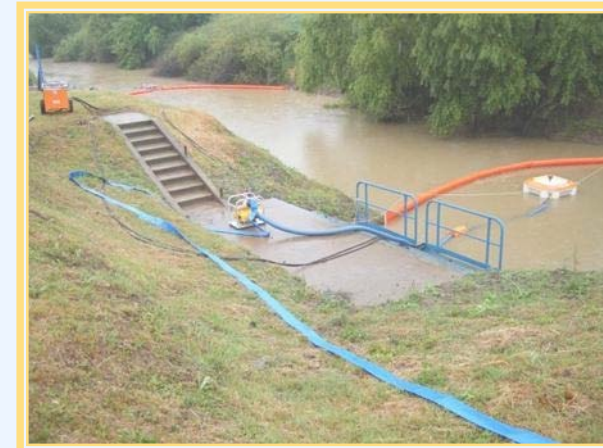
Practical bilateral exercise A practical bilateral exercise was organised in the framework of this project to test the plan and operational procedures. On the left, a water analysis in Oradea (RO), on the right, Pocsaj intervention site fully equipped with boom, skimmers, mobile pump and tanks (HU).
